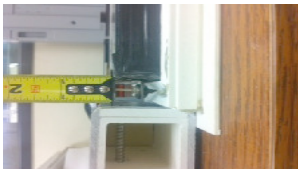
Correct Glazing Tape Compression
