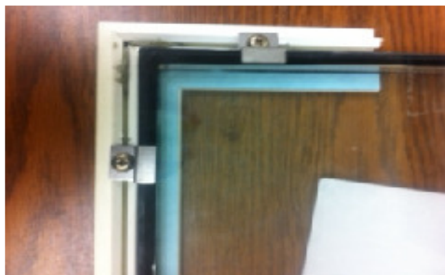
Security Screw Installation
